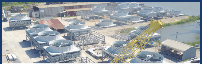
INDUSTRIAL MODULE YARD
